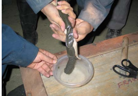
Squeezing the resin out from a two-compartment tube.
