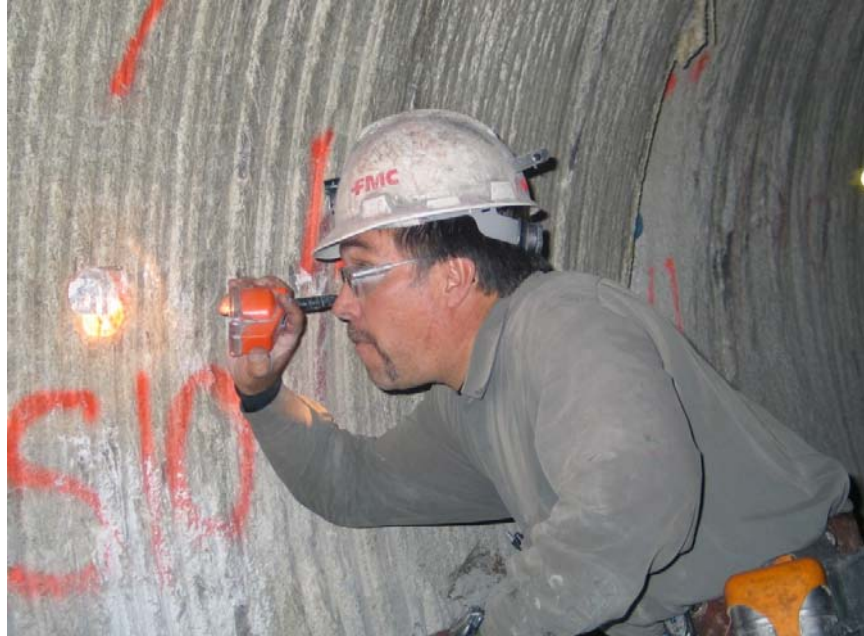
Sensor holes were carefully cleaned and inspected prior to sensor installation.
