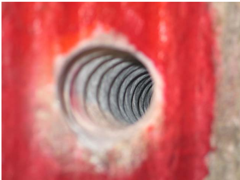
A thoroughly cleaned and dust-free sensor hole.
