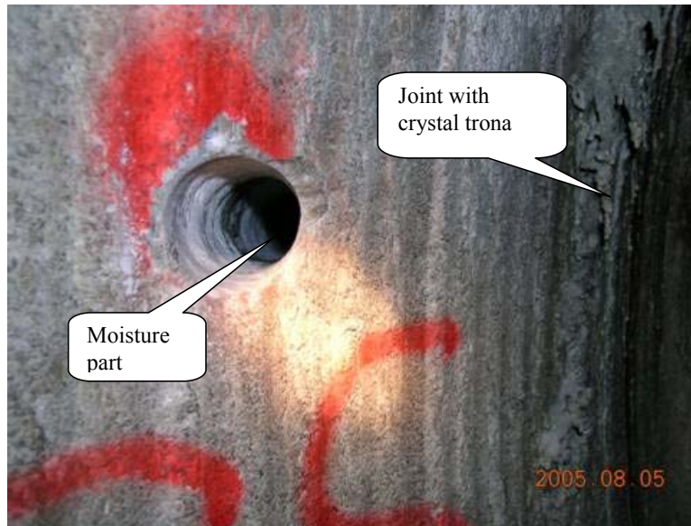
Figure.8.3 A trace of moisture showed in Sensor hole S5.
