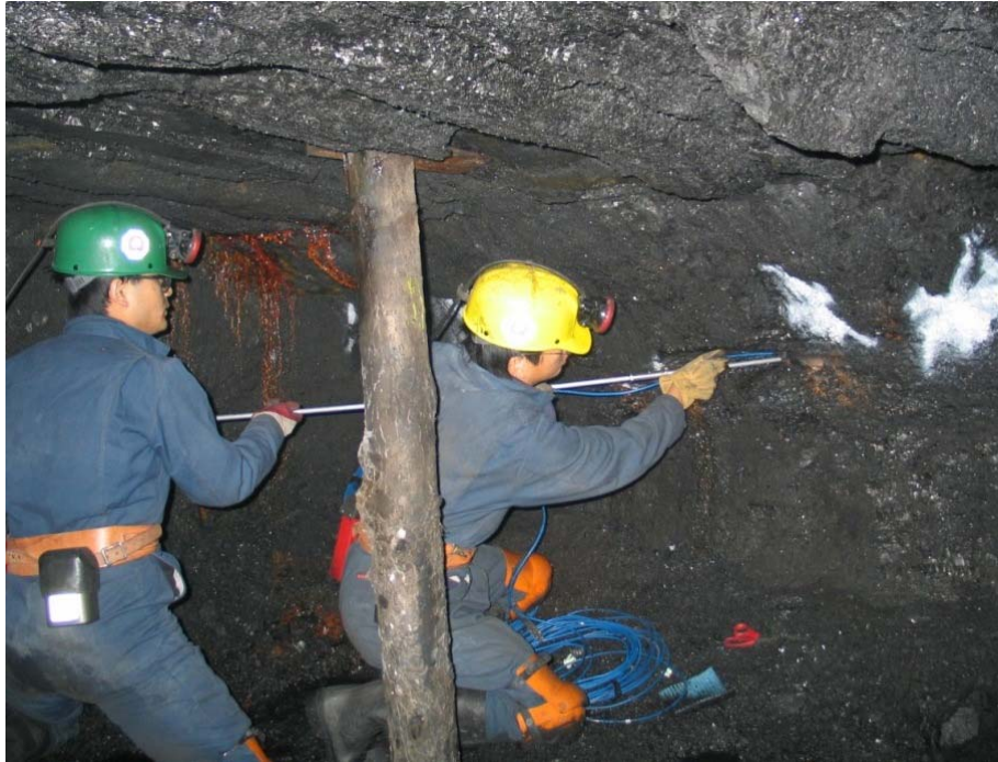
Figure 5.5 Sensor installation at the demonstration site.
