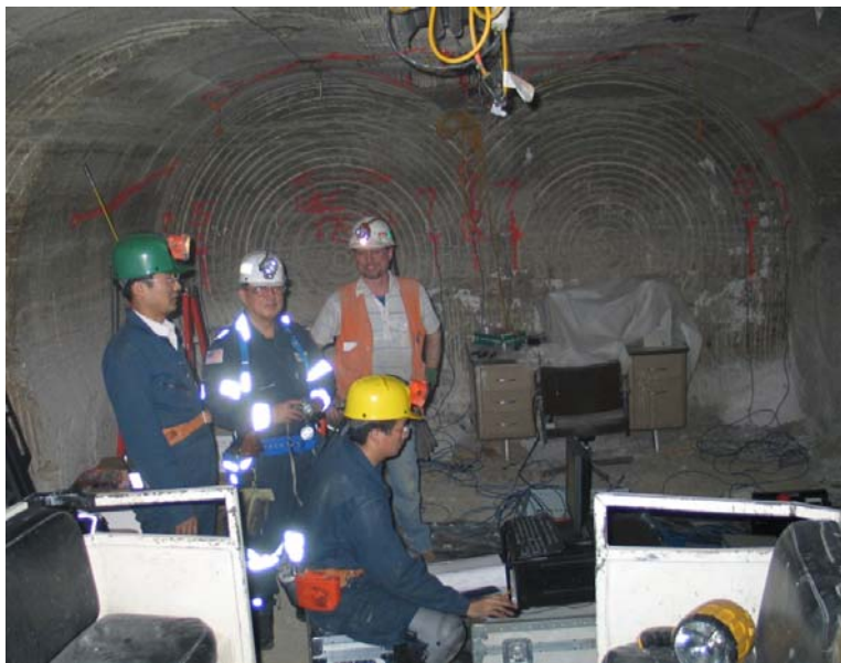
Figure 6.6 Field station for transmission survey, where the sensor holes were drilled at the face of the entry and the collar locations were marked by the vertical red lines.
