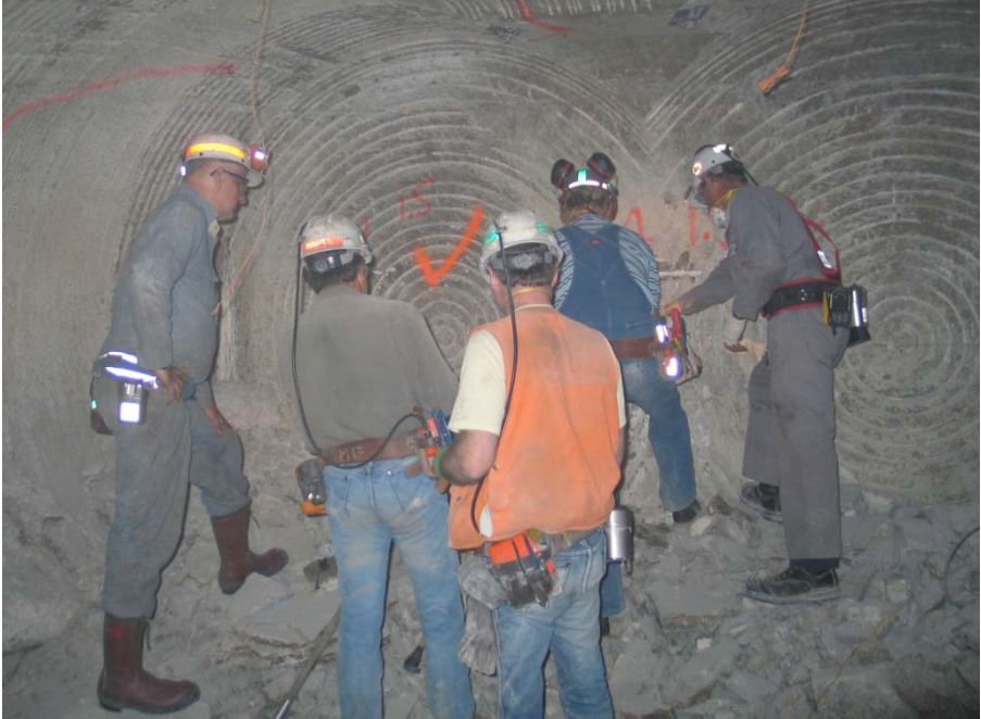
A scene at a blasting site.
