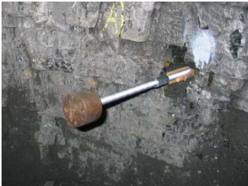
Figure 2.24 A Simple Mechanical Impact System (SMIS) installed in a coal pillar.
