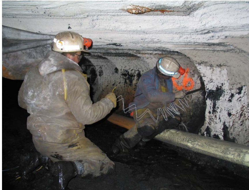
Figure 9.11. Setup the explosive for hole R6.
