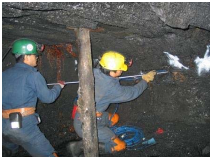
Figure 2.3 Installation of a retrievable sensor at the Harmony Mine.
