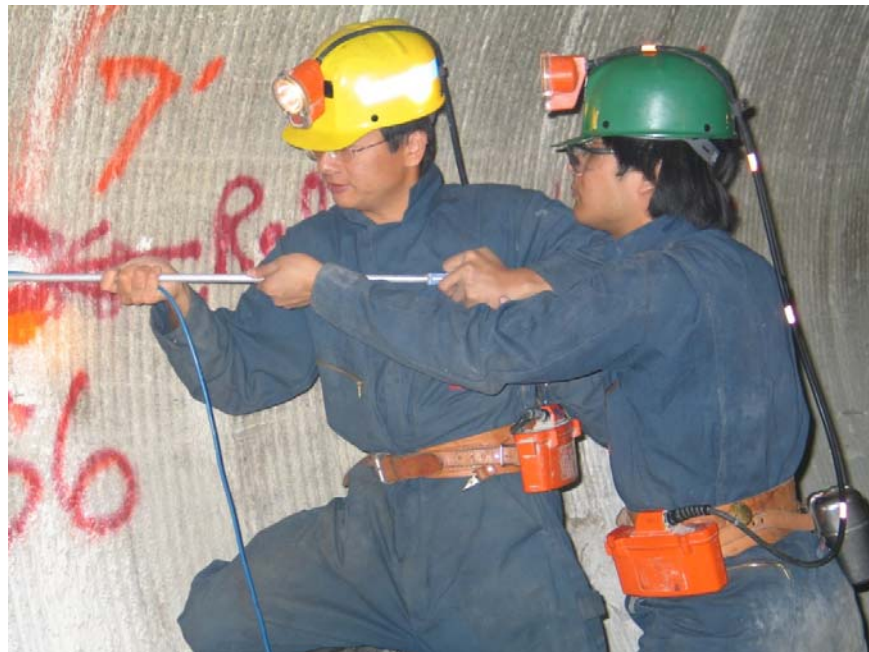
Sensor installation.
